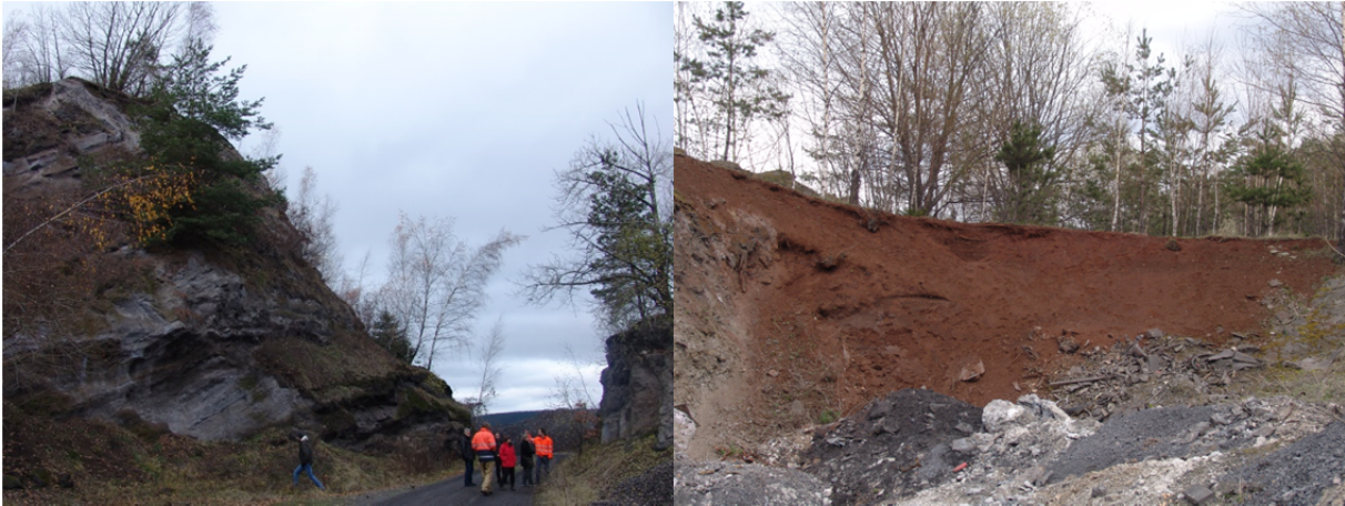
Fig. 3.5: Field impressions of the “Plateau 312”: View through the “Canyon” - a structure mainly formed of historic blast furnace slag - in northern direction (left), the eastern converter (dedusting) sludge basin (right).
