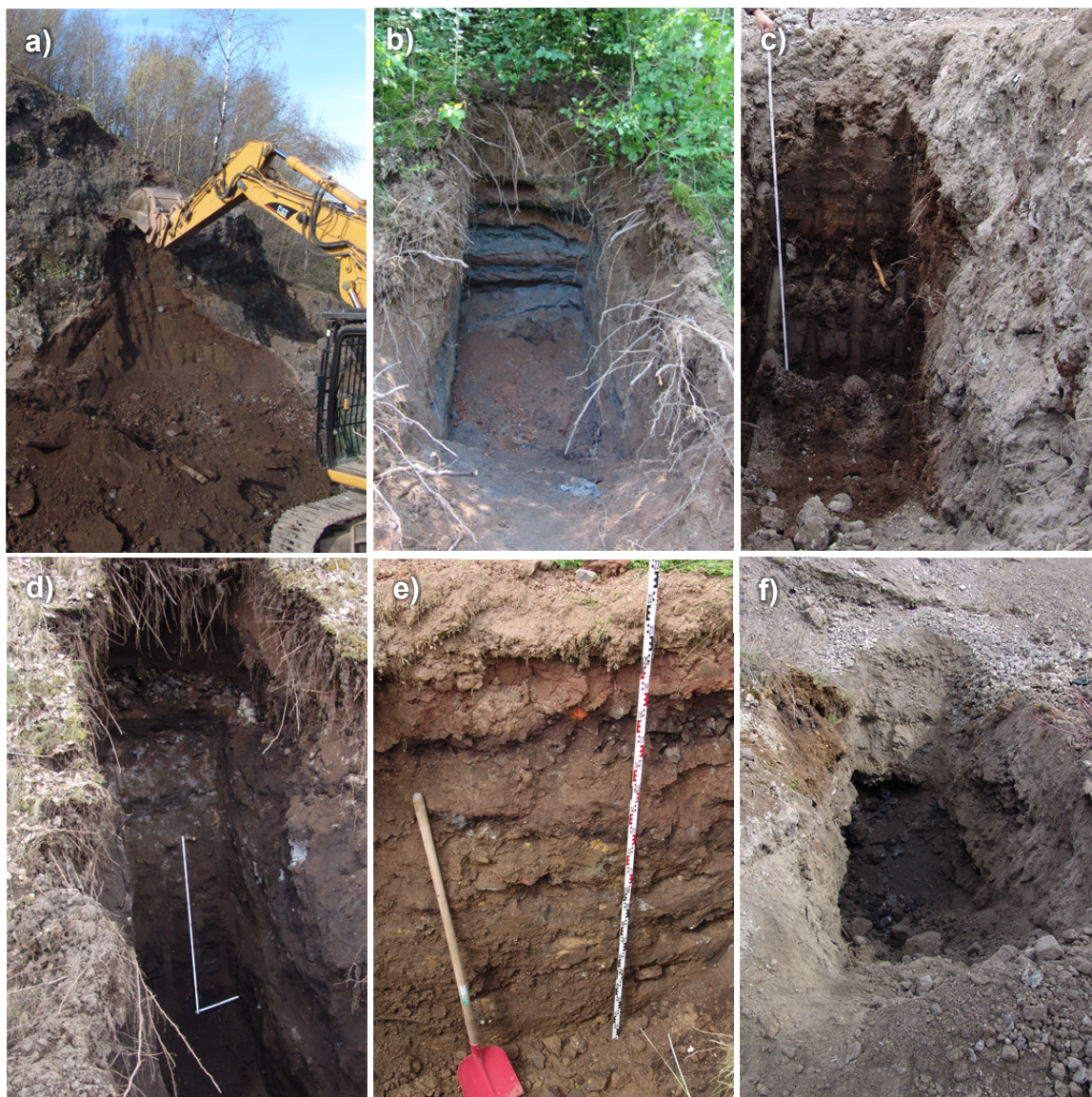
Fig. 4.3: Excavator prospectings: a) in the “Canyon”, b) close to the former “Sinterhang”, c) in the “Teich-Teich”, d) at the eastern part of the Plateau 312, e) at the Plateau 274 and f) at the western part of the “Hochhalde”.
