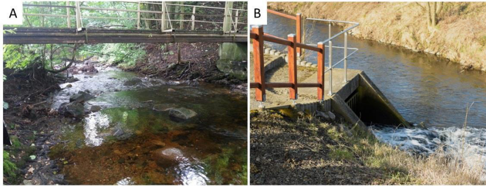
Figure 5.2: During the sampling campaign in 2014: A) Sampling location 5: ‘Braunes Wasser’ major tributary in the mountainous region, B) 29: inflow from WWTP II c) 33: Reconstruction zone: overflow collecting groundwater from the gravel pit
