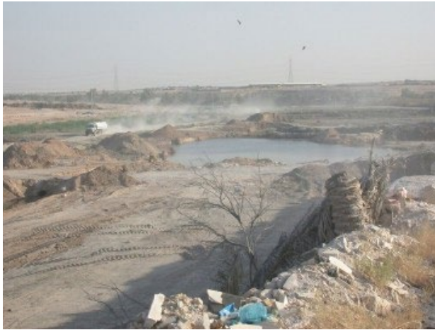
Fig. (42) Wadi Hanifah location before construction,
