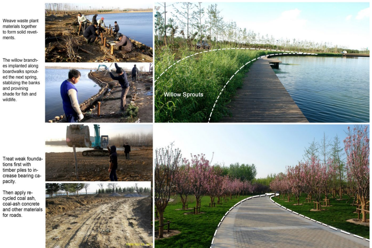
Fig. (48) The lakefront: was stabilized, load-bearing capacity was increased, and roads were constructed using waste plant materials and coal ash, Source: LPS-CSB- 494, 2012; Beijing Tsinghua Urban Planning & Design Institute; Biennal, An, Y., et al., 2014
