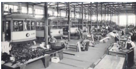
Fig. (118) Former Transit Maintenance facility, Source: Psomas, 2014
