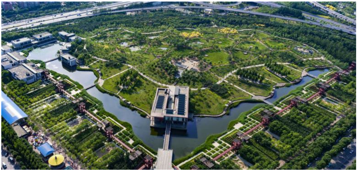
Fig. (68) Bird-eye view of the park, Source: World-Architects, 2013
