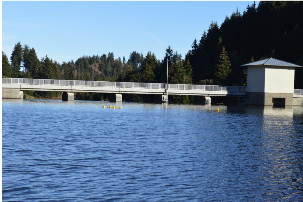
Photo: Rappbode pre-dam wall showing deep sampling point (group of buoys on the left). Photo by Tallent Dadi
