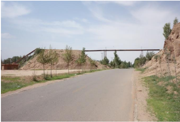
Figure 3.4 A pump house and canal are built to lift water from the primary surface water canal to elevated land
