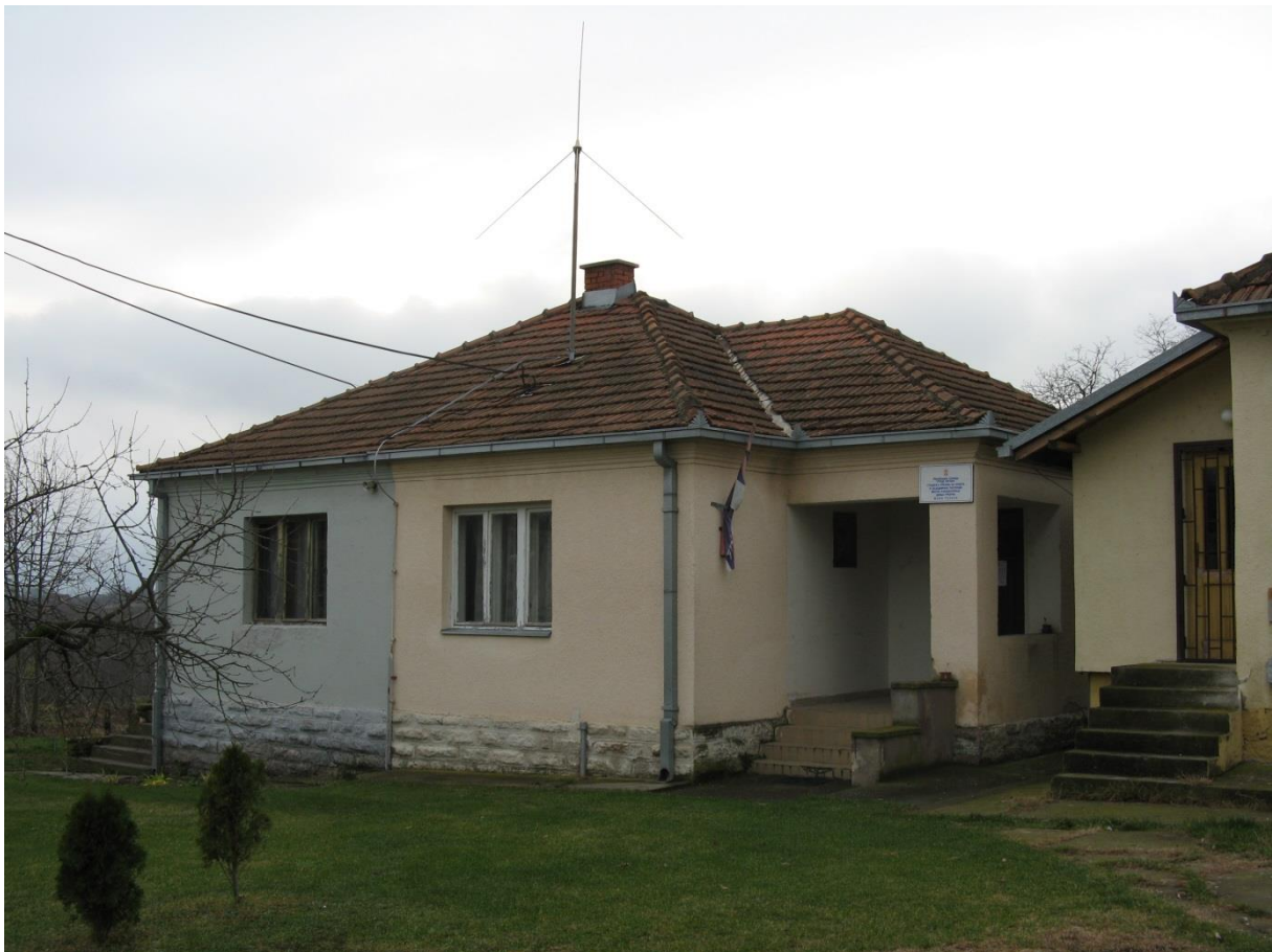
Figure 4: The Local Council building
