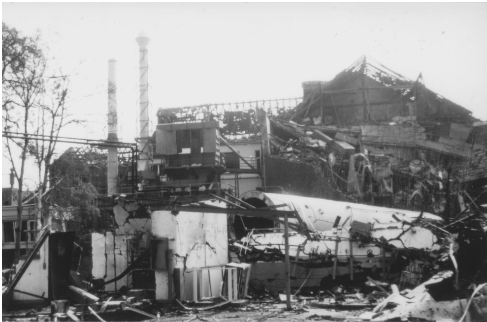
Figure 2.1: The explosion of a hydrogen storage tank destroyed big parts of a factory, causing immense economic costs [8].
