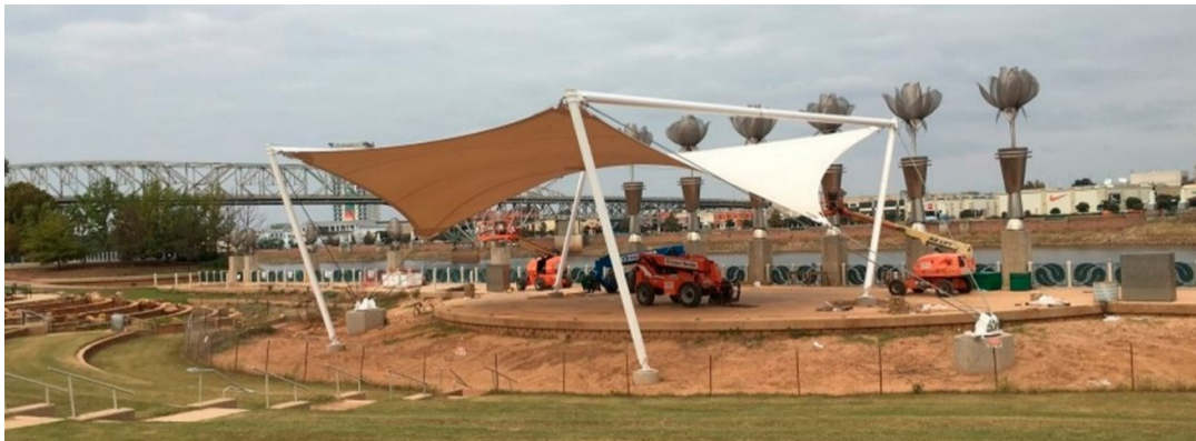
Figure 5.3 Steel structure with tensile fabric, done by Birdair, USA
