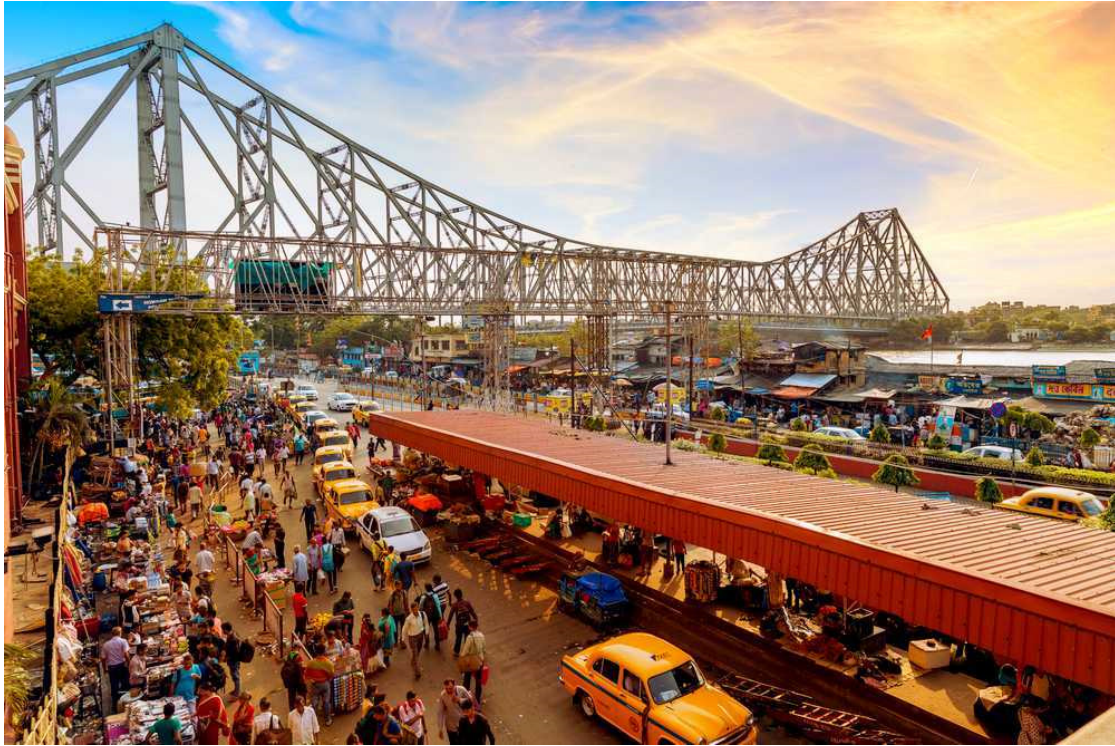
Figure 2.12 Howrah bridge, Kolkata
