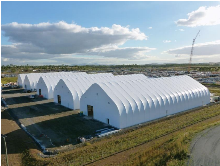
Figure 3: Examples of Keder style membrane buildings, photo courtesy of Norseman Group Ltd.
