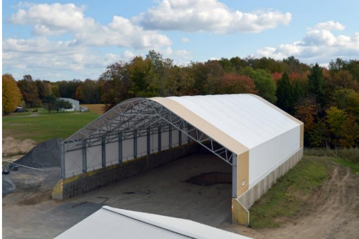
Figure 7: I-beam Sidewall style, photo courtesy of Norseman Group Ltd.
