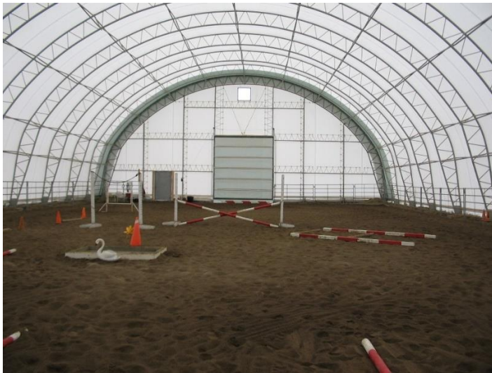
Figure 6: The double truss building style, photo courtesy of Pembina Valley Canvas.
