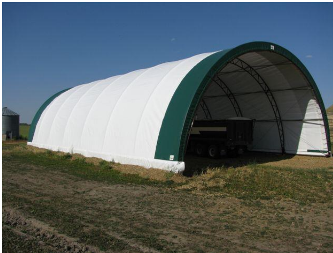
Figure 2: Example of a single cover steel framed building, photo courtesy of HiQual Alberta.
