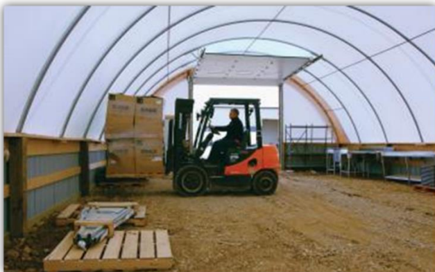
Figure 5: Single Truss building style, , photo courtesy of Norseman Group Ltd.
