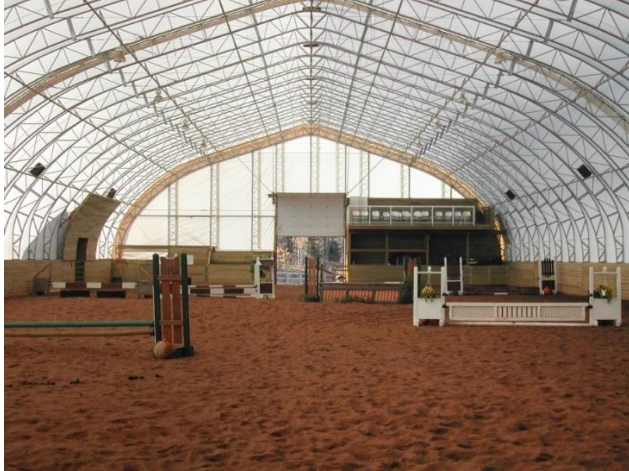
Figure 4: Mono covers joined by Keder extrusion, photo courtesy of Les Industries Harnois.
