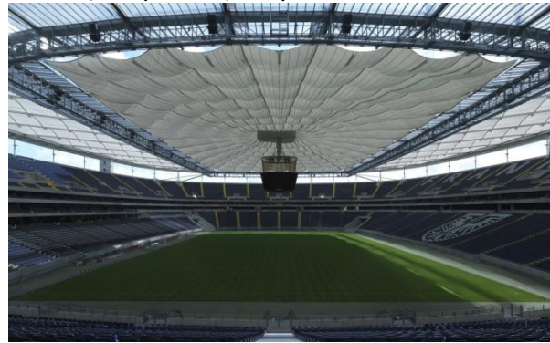
Figure 10: Commerzbank-Arena Frankfurt in almost deployed position, Frankfurt, Germany (Schlaich Bergemann Partner, 2006)
