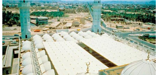
Figure 8: Quba Mosque toldo shading in deployed position, Madinah, KSA (SL Rasch, 1987)
