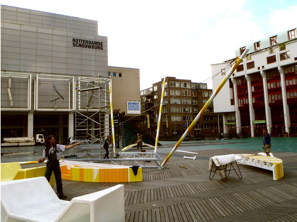
Fig. 10.8: Raising the masts
