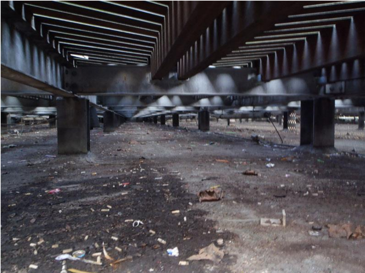
Fig. 7.13: Flore covered with bitumen
