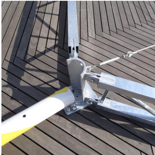
mastholder installed
