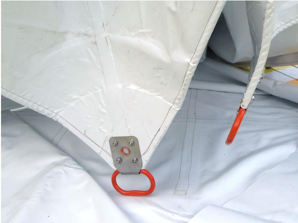
Fig. 8.10: guy cable connections
