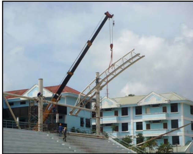
ERECT 1/4 TRUSS @ X1
