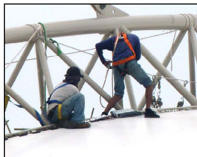
FABRIC TENSIONING
