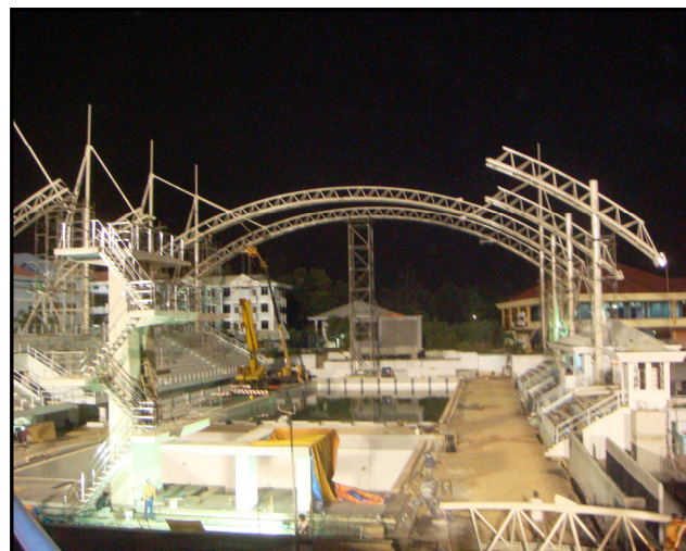
ERECTED TRUSS @ X2
