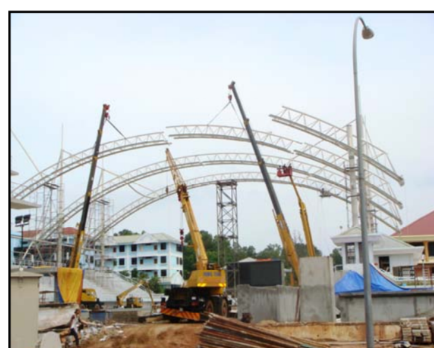
ERECTING TRUSS @ X3
