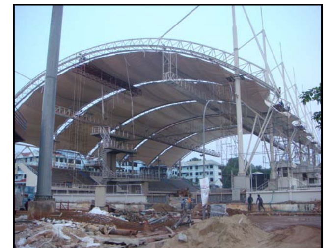
5 TH FABRIC PANEL INSTALLED
