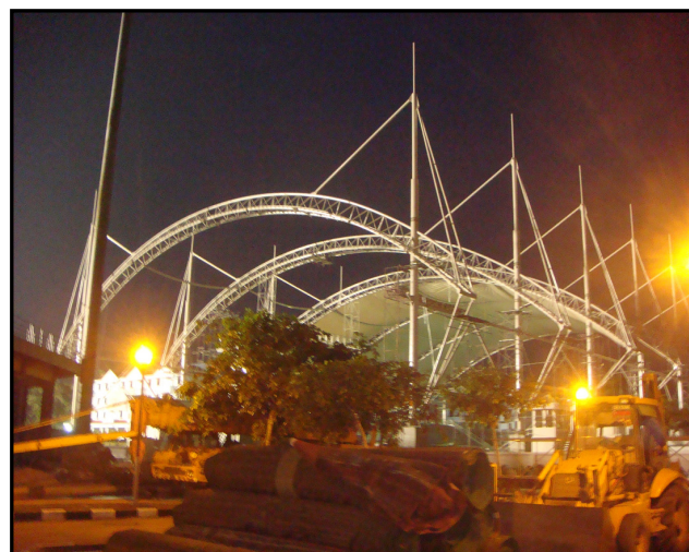
ERECTED TRUSS @ X6
