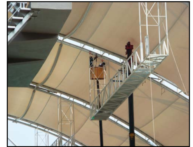
ERECTING CATWALK
