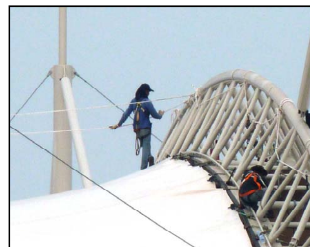
WARP TENSIONING
