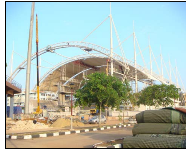
ERECTED TRUSS @ X6
