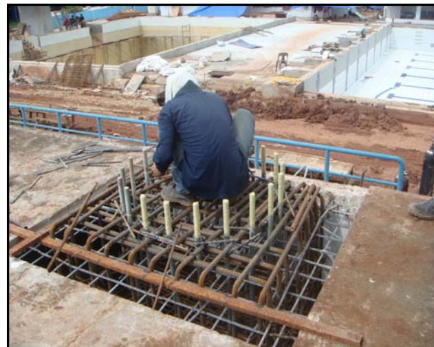
INSTALL HD BOLT
