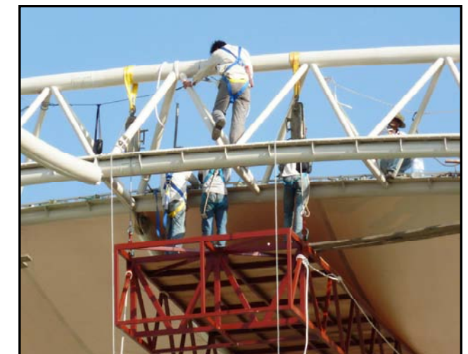
FABRIC TENSIONING
