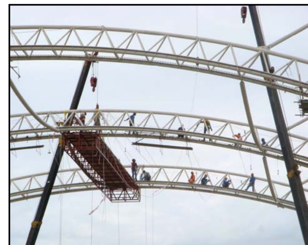
FIXING HOLDING ROPES
