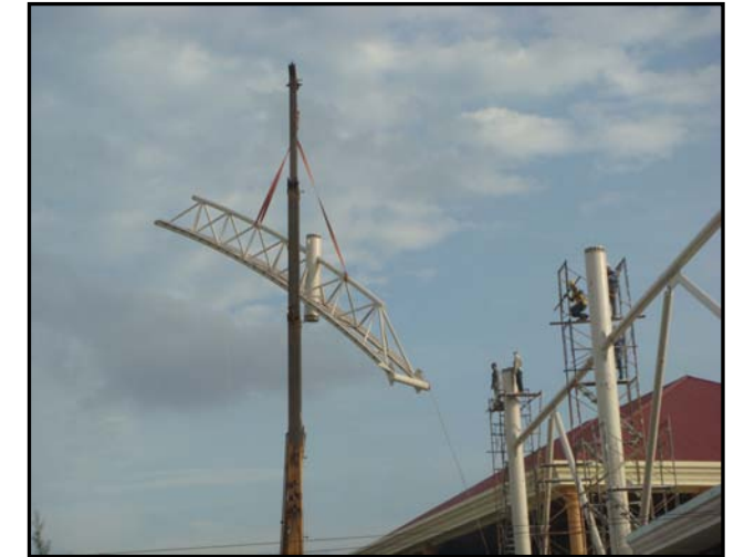
ERECT 4/4 TRUSS @ X1
