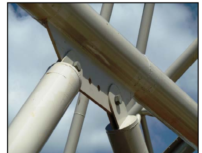
COLUMN BRACING CONNECTION
