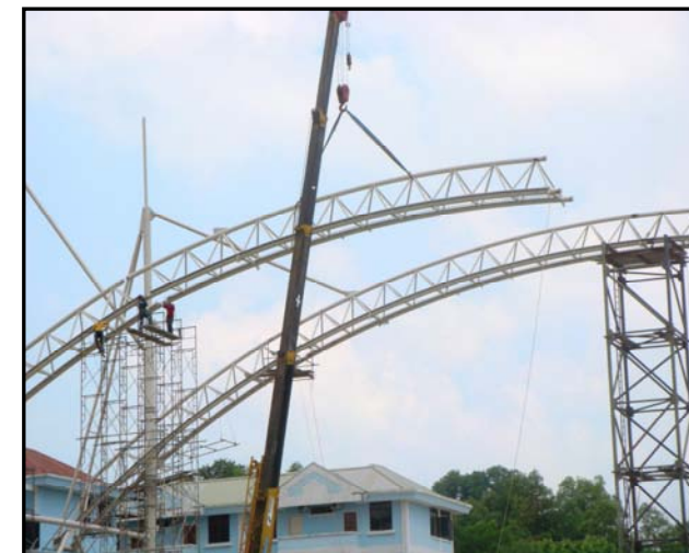
ERECT 2/4 TRUSS @ X2
