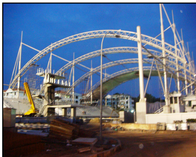
ERECTED TRUSS @ X5
