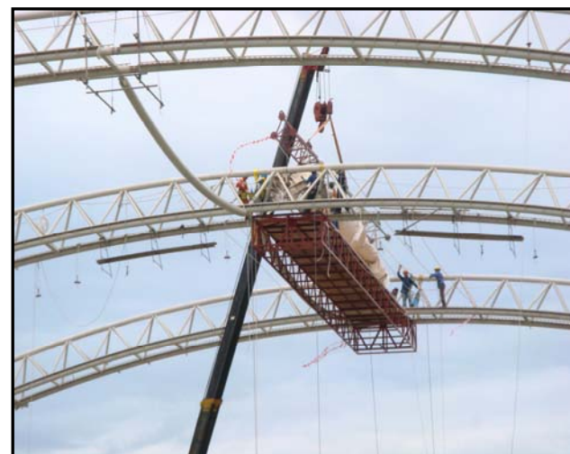
1 ST PANEL ON PLATFORM
