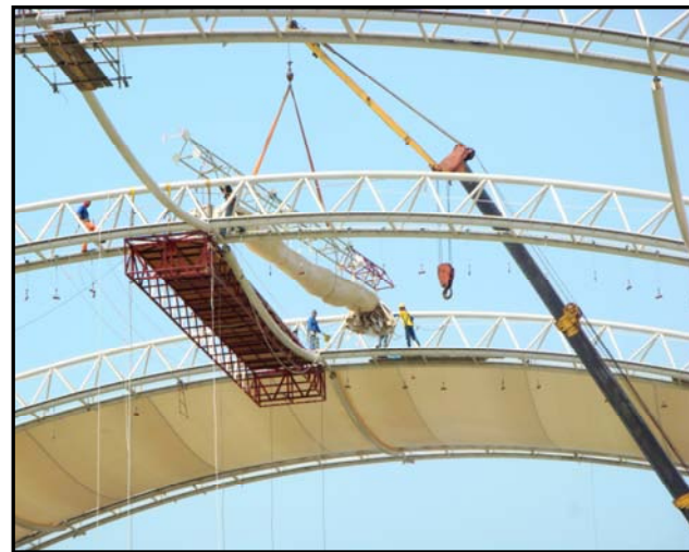
INSTALLING 2 ND FABRIC PANEL
