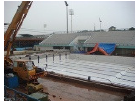
CRANE ACCESS BESIDE POOL
