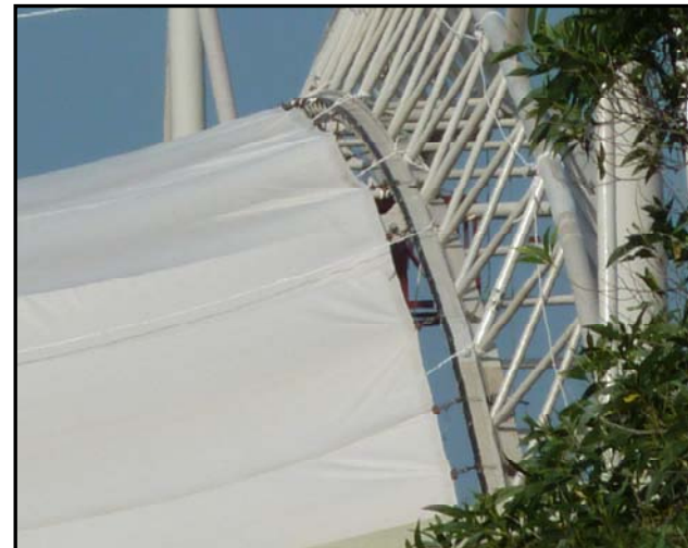
FABRIC TENSIONING
