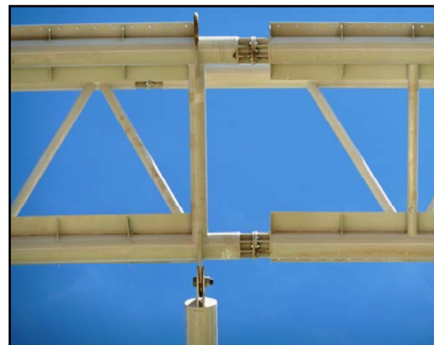
TRUSS FLANGE & TIE JOINT
