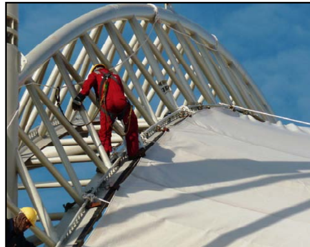
FABRIC TENSIONING
