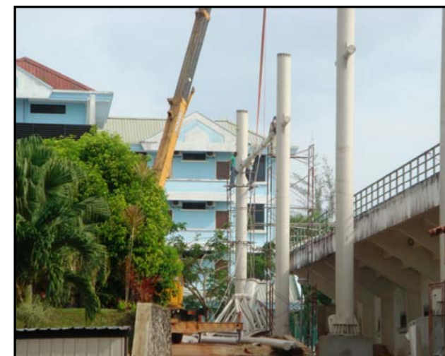
ERECT COLUMN TIE
