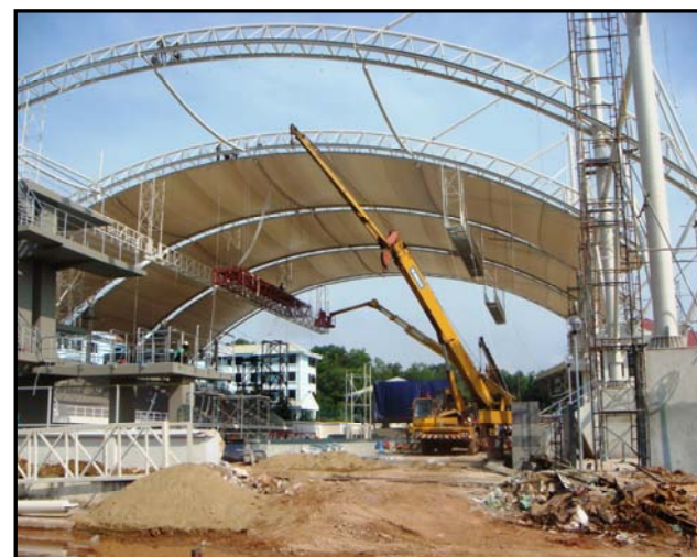
3 RD FABRIC PANEL INSTALLED
