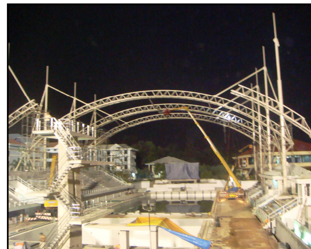
ERECTED TRUSS @ X3
