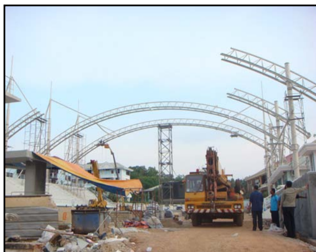
ERECTED TRUSS @ X2
