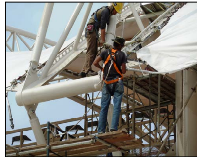
WEFT TENSIONING AT CORNER
