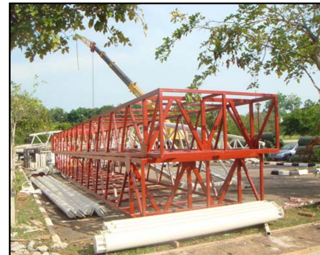
FABRIC ERECTION PLATFORM
