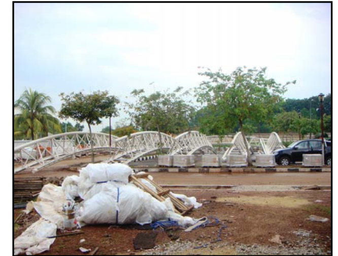
TRUSS STORAGE AT SITE
