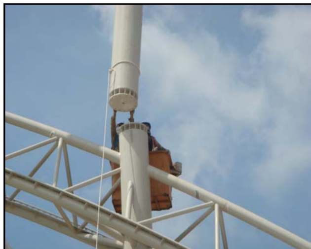
ERECT UPPER COLUMN
