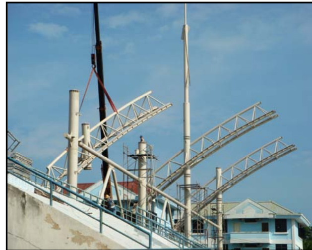
ERECT UPPER COLUMN
