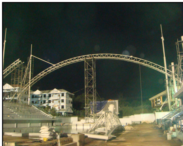
ERECTED TRUSS @ X1
