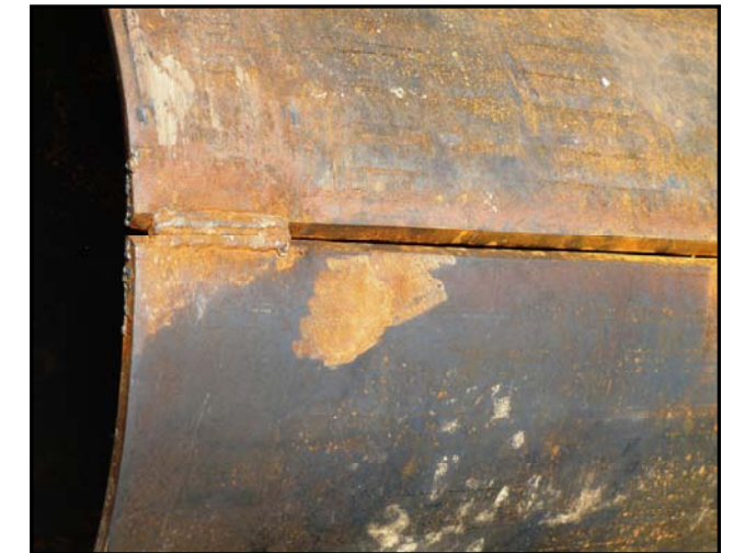
WELDING PREPARATION FOR COLUMN
