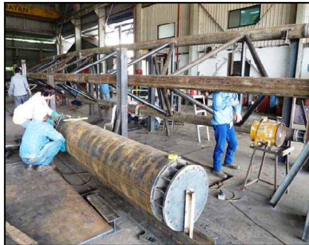
TRUSS & COLUMN FABRICATION
