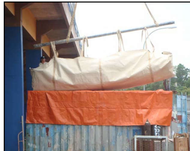
FABRIC PANEL AT SITE
