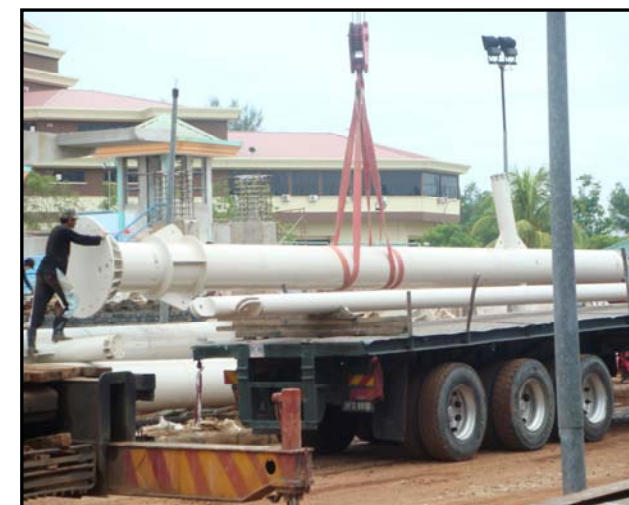
UNLOADING OF COLUMN
