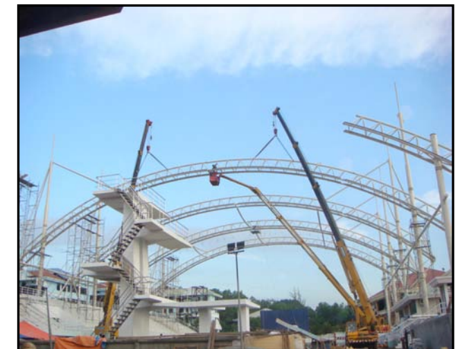
ERECTING TRUSS @ X4
