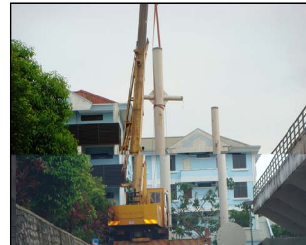
ERECT LOWER COLUMN
