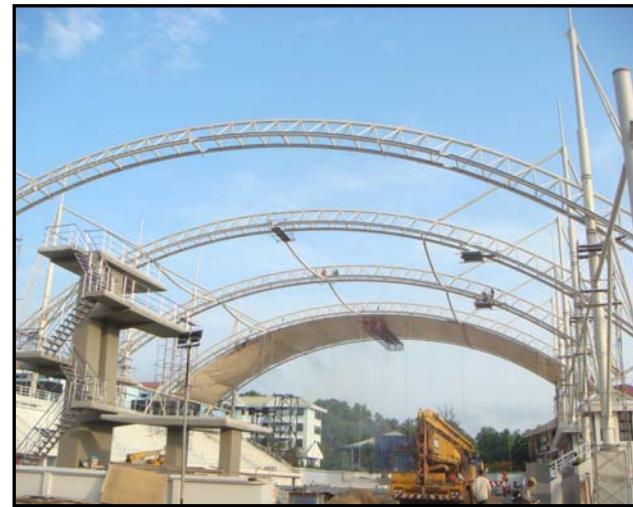
ERECTING TRUSS @ X5
