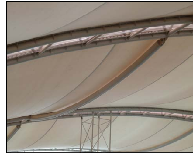
TIE BEAM CLEARANCE
