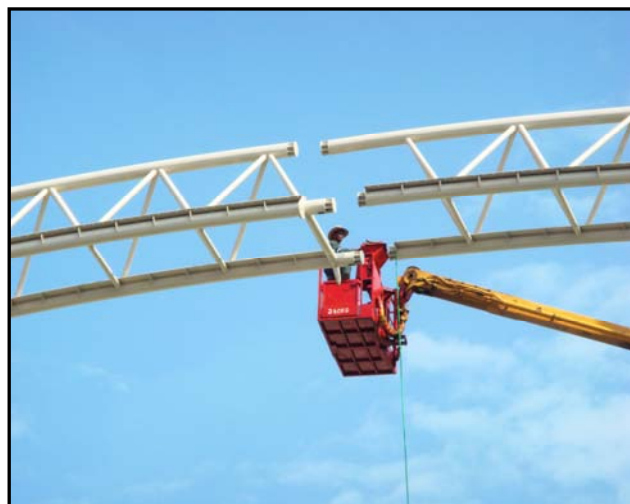
TRUSS FLANGE CONNECTION
