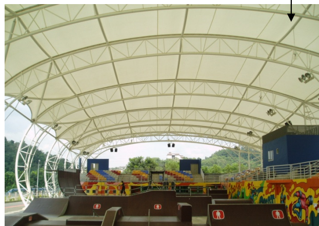
TRUSS TIE SYSTEM TO BUKIT KIARA X-TREME SPORT COMPLEX
