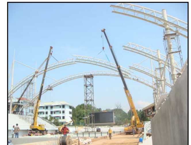
ERECT 3/4 TRUSS @ X2
