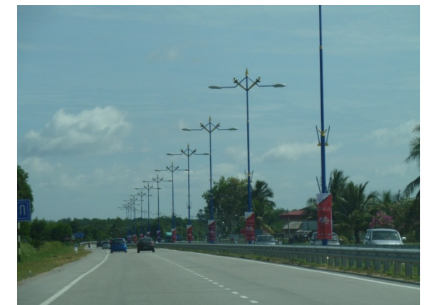
MORE BANNERS ALONG ROAD TO SITE
