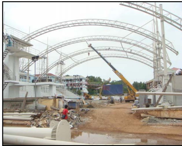
ERECTED TRUSS @ X4
