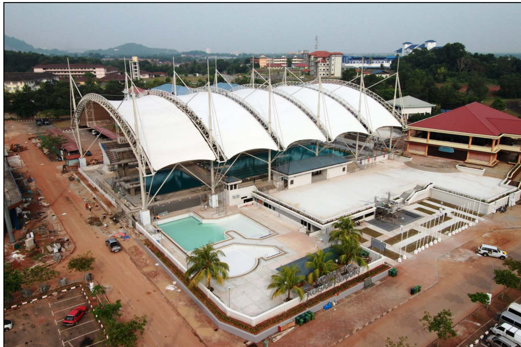
AERIAL VIEW – PHASE 1 COMPLETION
