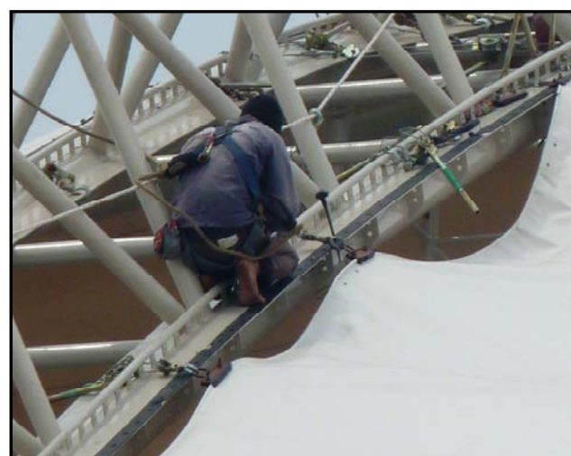
WARP TENSIONING
