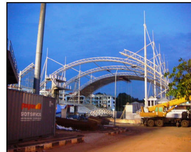
ERECTED TRUSS @ X4
