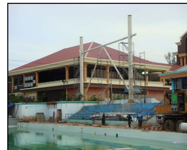
ERECT COLUMN TIE
