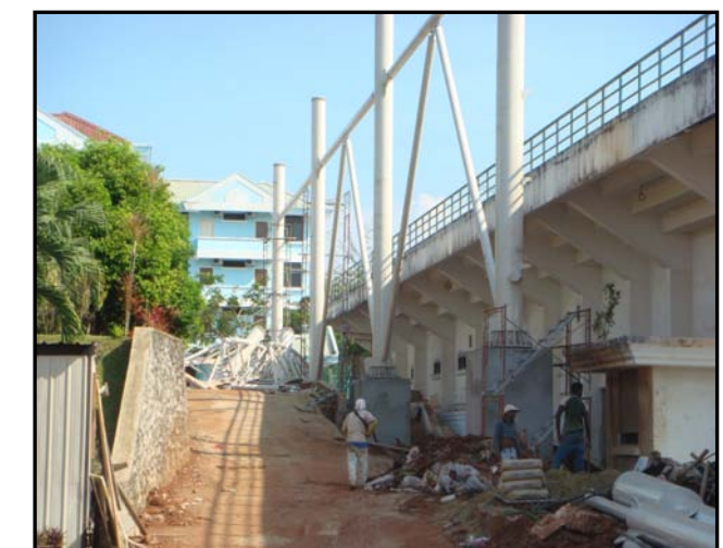
ERECTED COLUMN TIE
