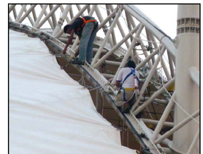
WARP TENSIONING
