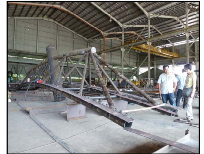
TRUSS WITH COLUMN
