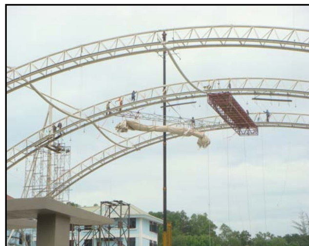
LIFTING 1 ST FABRIC PANEL
