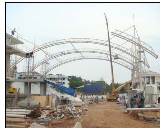
ERECTED TRUSS @ X3
