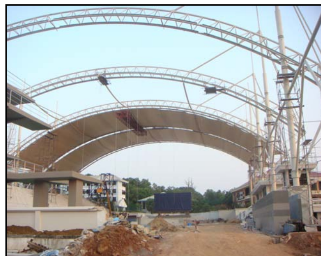
2 ND FABRIC PANEL INSTALLED
