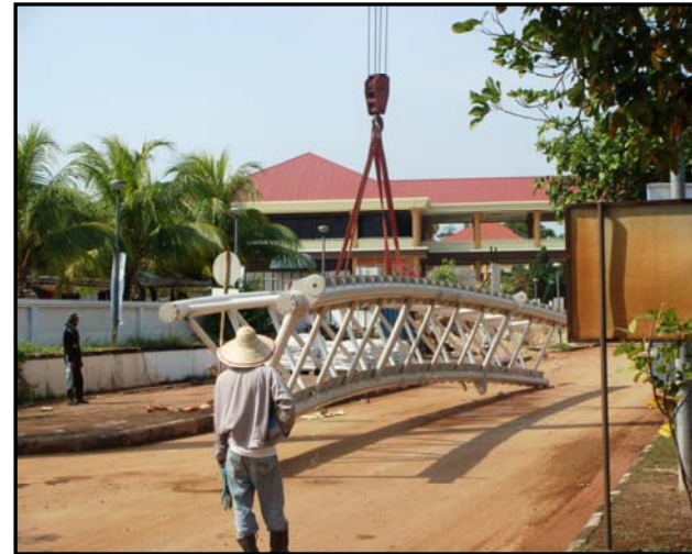
UNLOADING OF TRUSS
