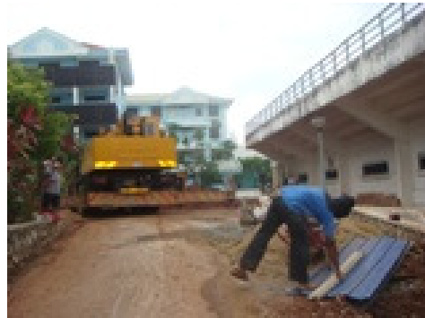
CRANE ACCESS BESIDE EXISTING HOSTEL BLOCK AT REAR OF SITE
