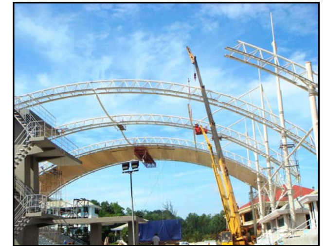
1 ST FABRIC PANEL INSTALLED
