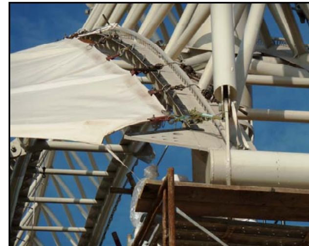
FABRIC TENSIONING
