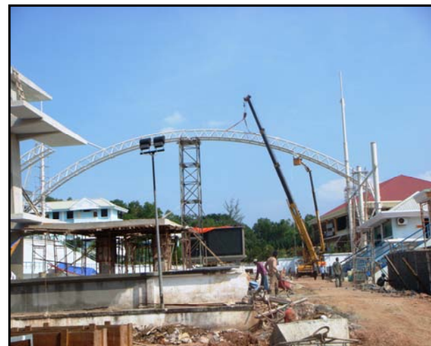
ERECT 3/4 TRUSS @ X1
