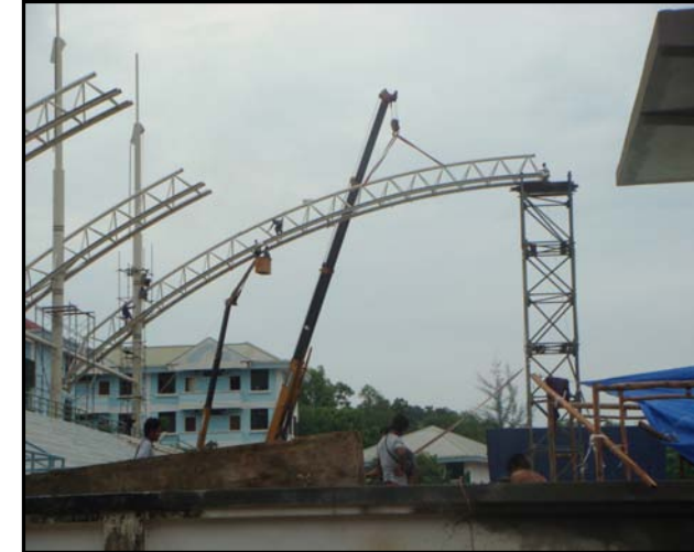
ERECT 2/4 TRUSS @ X1
