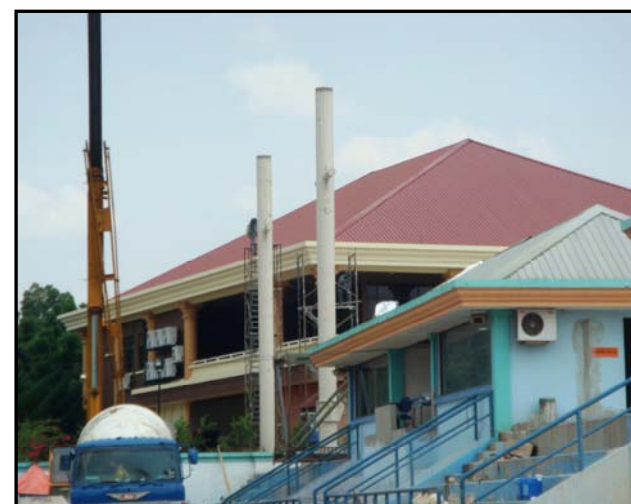
ERECT LOWER COLUMN
