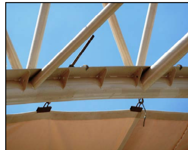
WARP TENSIONING
