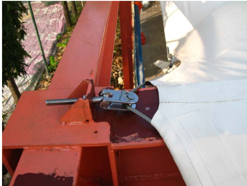
Figure 3.2 Boundary cables and Thread toggle
