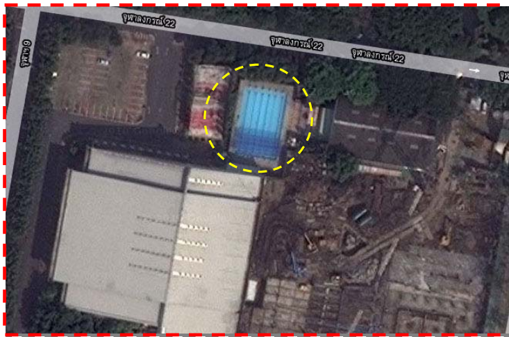
Figure 1.4 Arial view of the swimming pool
