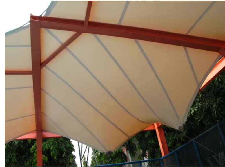
Figure 2.13 PVC coated polyester membrane
