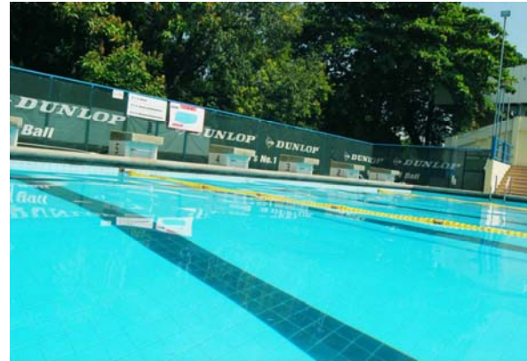
Figure 1.7 Existing condition of the swimming pool (on North wing)
