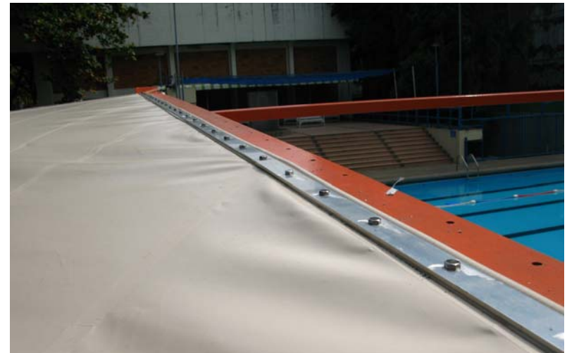
Figure 4.6 Clamping Plate Edge (II)
