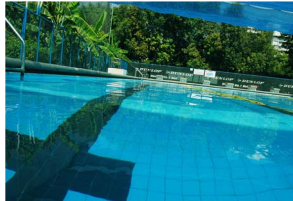
Figure 1.8 Existing condition of the swimming pool (on West wing)
