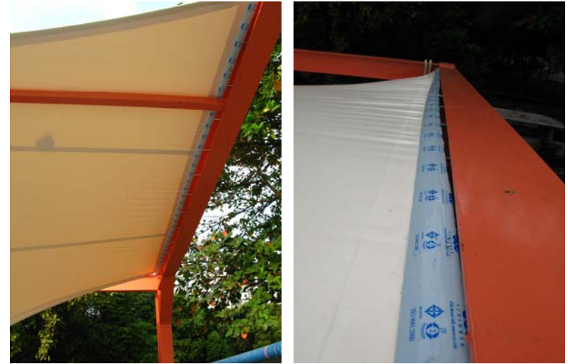
Figure 4.5 Clamping Plate Edge (I)
