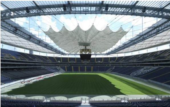
Figure 9: Commerzbank-Arena Frankfurt toldo shading in semi retracted position, Frankfurt, Germany (Schlaich Bergemann Partner, 2006)
