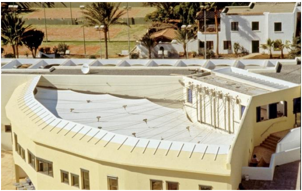
Figure 12: Robinson club toldo shading in deployed position, Canary Island, Spain (SL Rasch, 1999)
