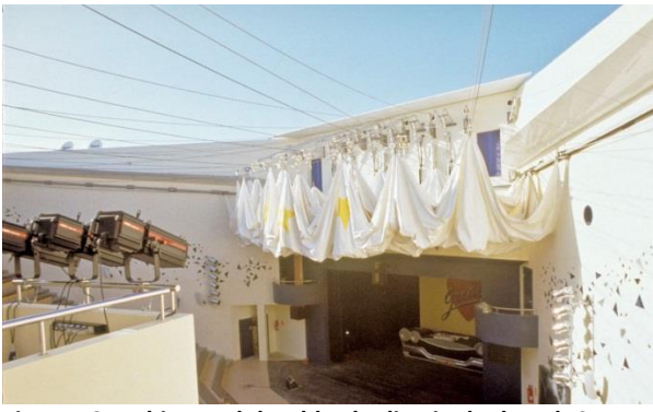
Figure 13: Robinson club toldo shading in deployed, Canary Island, Spain (SL Rasch, 1999)
