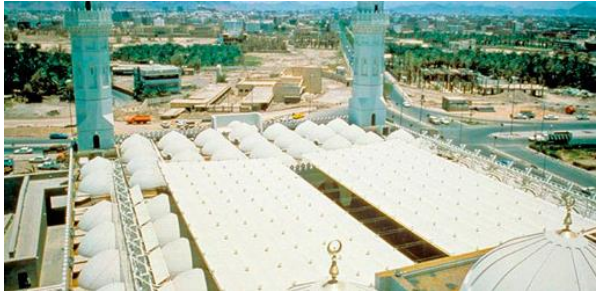
Figure 8: Quba Mosque toldo shading in deployed position, Madinah, KSA (SL Rasch, 1987)
