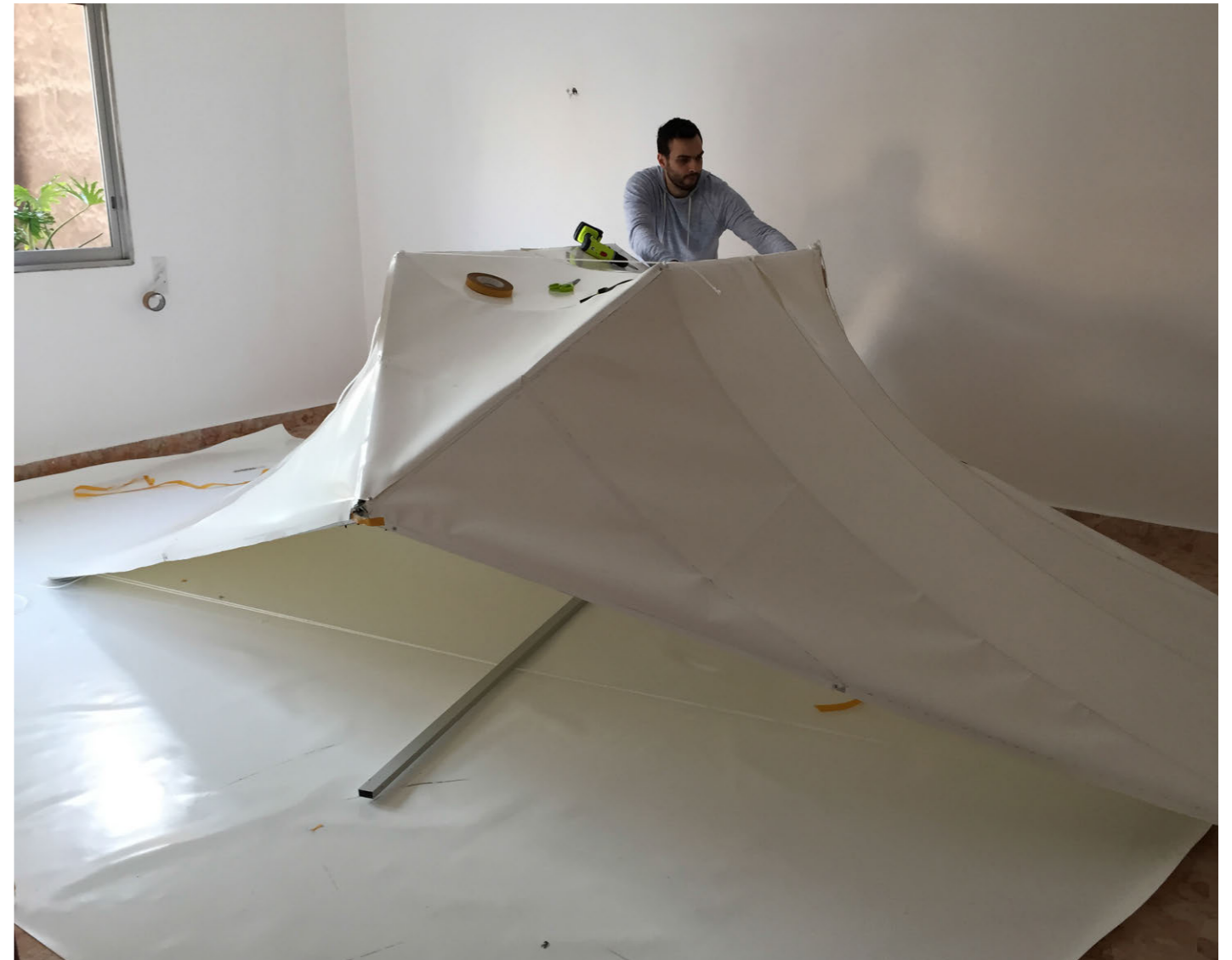
Pattern assembly before tensioning with the lower cable
