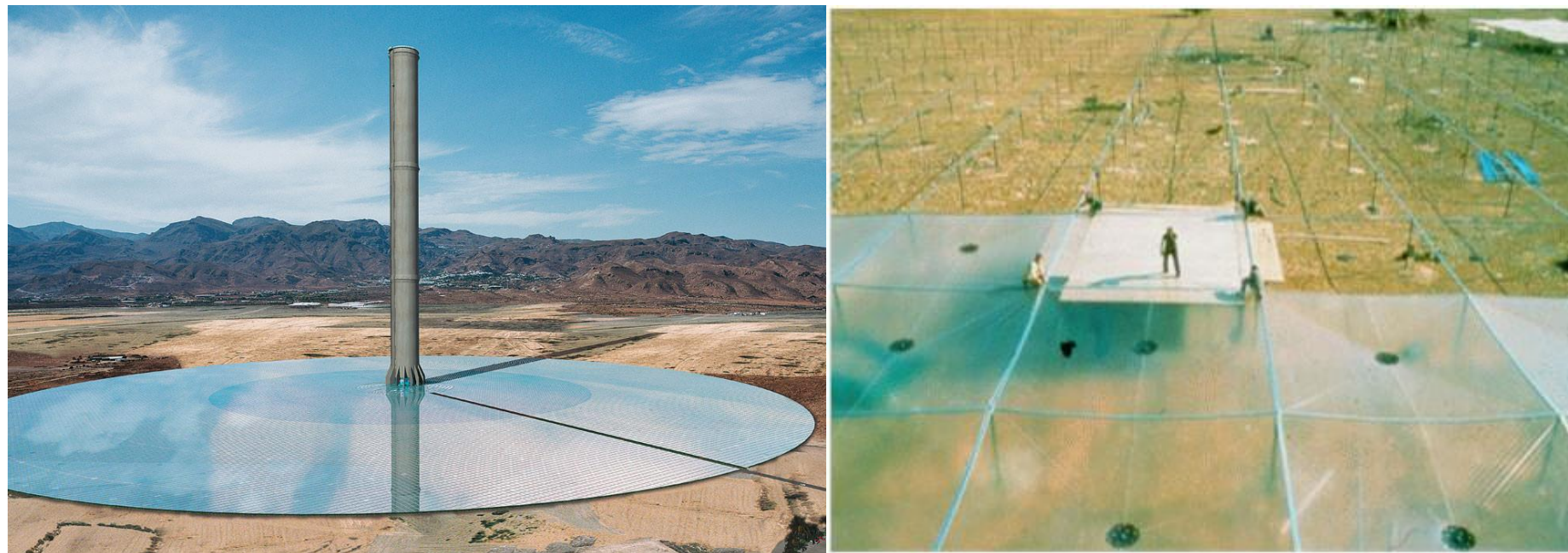
Figure 18 –Solar Updraft Tower (left) and ETFE film for solar updraft tower in Manzanares, Spain (right) (Copyright: Schlaich Bergermann und Partner)
