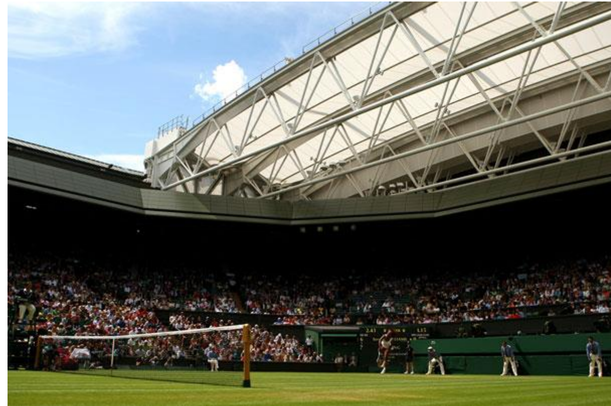
Figure 7 – Centre Court Wimbledon – Retractable Roof (Source: www.nytimes.com )
