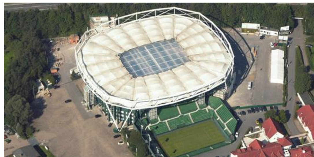
Figure 3 - Gerry Weber Stadium with ETFE Retractable Roof (Source: www.skyscrapercity.com )
