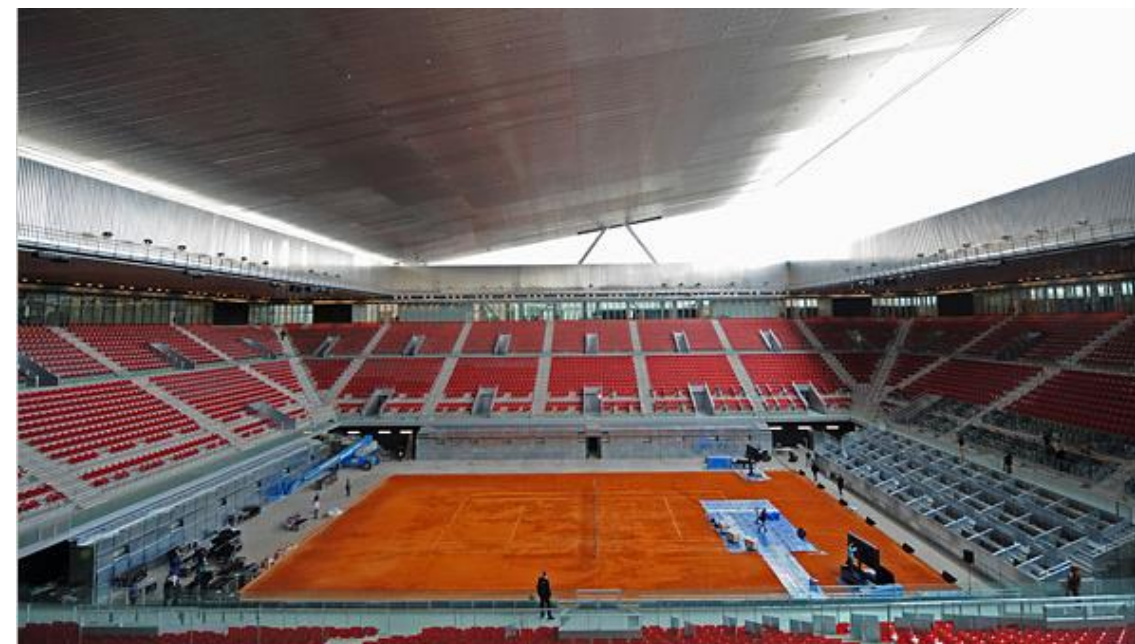
Figure 6 – Magic Box Stadium in Madrid – Retractable Roof (Source: www.nytimes.com )
