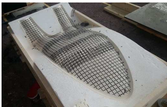
Fig. 31: Laying of carbon reinforcement mesh
