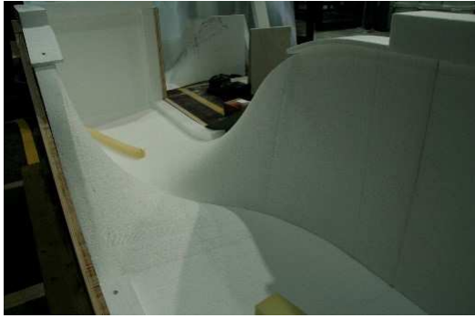
Fig. 23: Assembly of the Styrofoam mold parts
