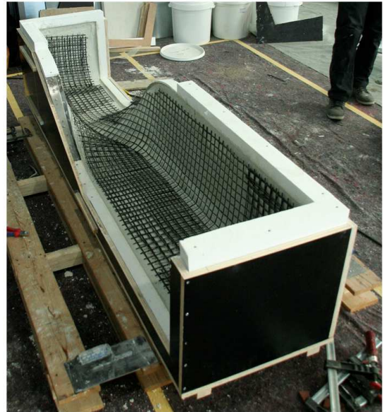
Fig. 26: Laying of carbon reinforcement mesh
