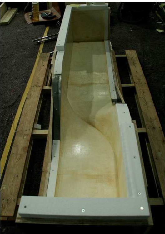
Fig. 25: Applying formwork oil as release agent
