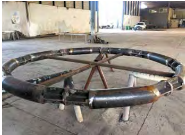
Ring beam as supporting structural element Source: Big Span Structures
