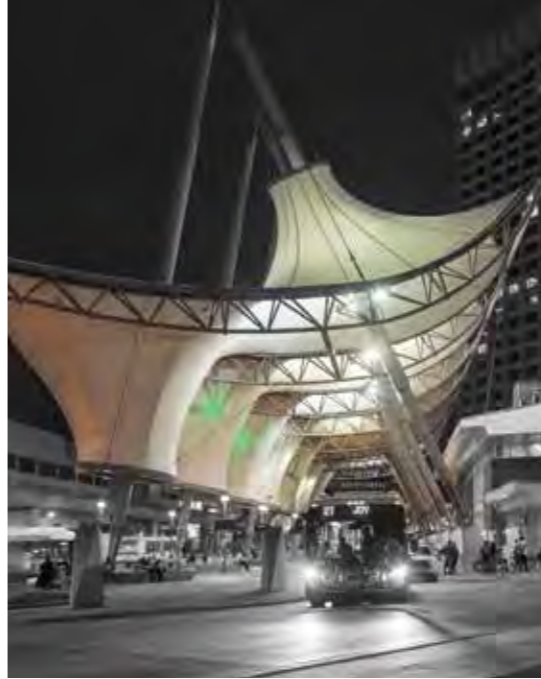
Above: Model with Formfinder Software Tensile Fabric Patterning (IxCube) Rosa Parks Transit Center, Detroit (USA) Architecture: FTL Design Engineering Studio
