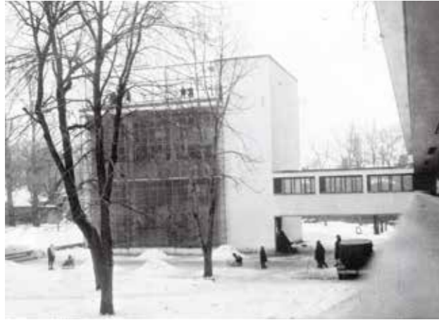
The Narkomfin Communal House was built as part of the state-run Soviet Experimental Building Programme (1928) on the Moscow Garden Ring. In the glass pavilion, in addition to communal facilities, there was also a temporary kindergarten. Photo: Archive of families Miljutin and Ginzburg, Moscow
