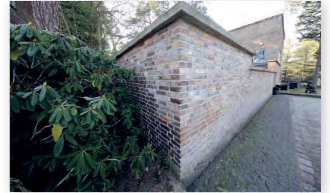
Concrete cover plates with an overhang accentuate the strong horizontal appearance of the building.
