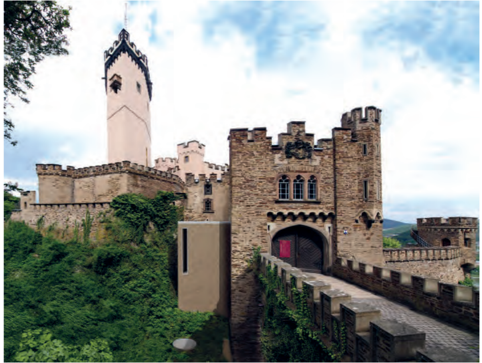
To enable wheelchair users to visit, an accessibility plan was devised and a lift installed in a washed brickwork tower erected next to the gatehouse. The renovated façade also demonstrates this successful reconciliation of preservation with progress. Picture: Natascha Meuser
