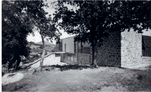
1 The entrance to the house is almost like a processional staircase. The building and landscape were meant to be experienced as one. Picture: Utzon Photos
