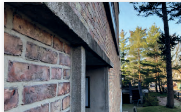
Horizontal concrete details run through the brick wall.
