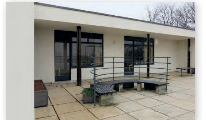
Travertine on the parapet and garden terrace with stairs
