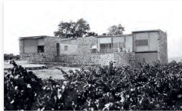
A narrow natural stone path runs in axis to the entrance. Picture: Le Corbusier Foundation
