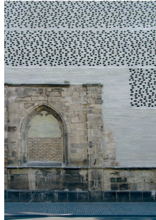
Peter Zumthor: Kolumba – Art Museum of the Roman Catholic Archdiocese of Cologne, 2007 Pictures: DOM publishers
