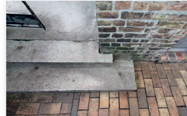
Concrete and brick dress walls and floors.
