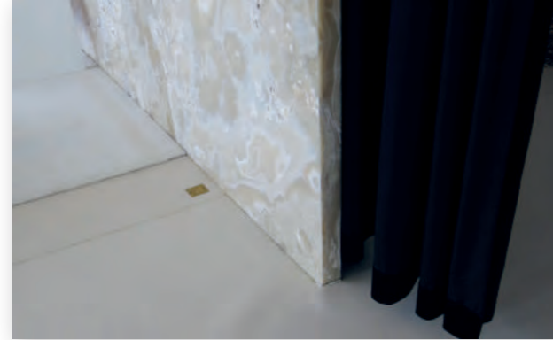
Jointless meeting of the linoleum and stone
