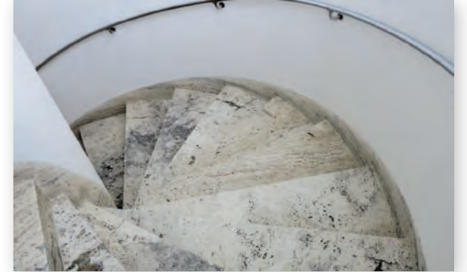
Travertine staircases with flush-walled skirting boards
