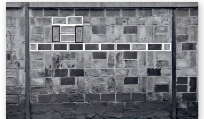
Concrete cover plates finish the brick wall with its bond pattern.
