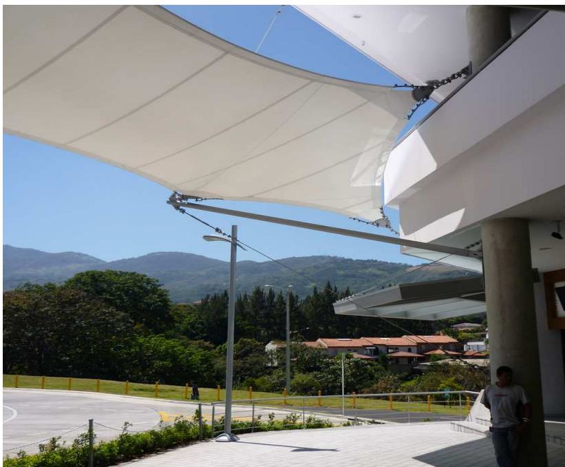
Fig. 88 Picture: View from below
