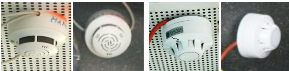
Figure 53 – Hekatron ORS 142 Rail and Fireduct S65
