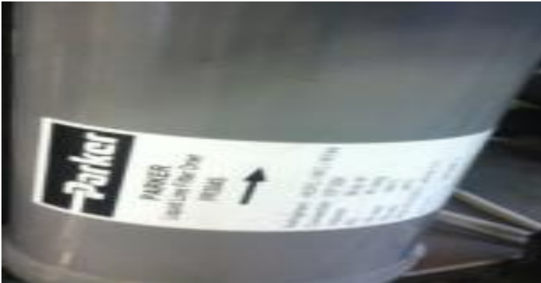
Abbildung 5.7: Liquid Line Filter Drier
