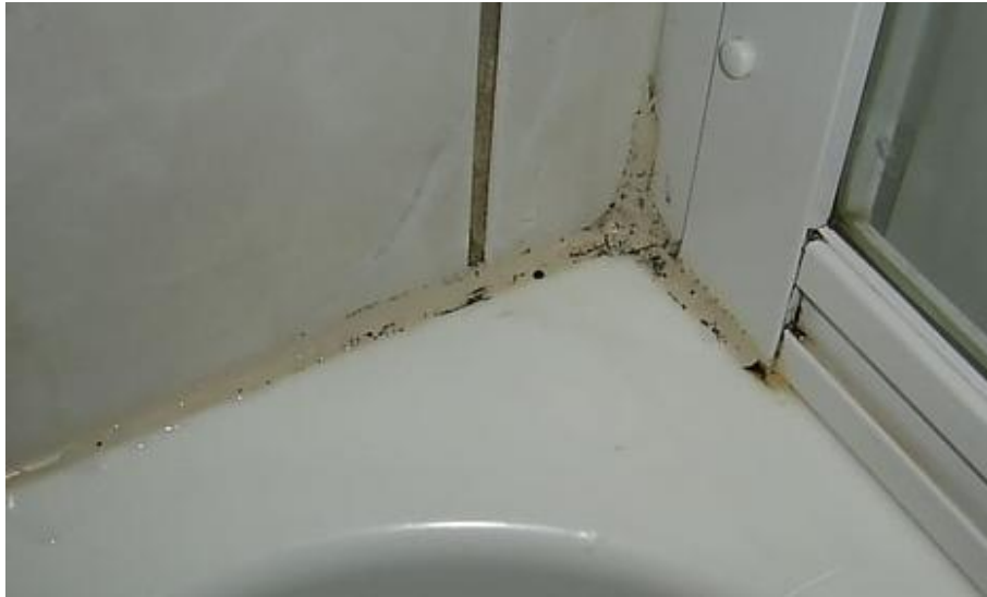
Fig. 14: Colonization of silicon seals by fungi in a shower tray [19]
