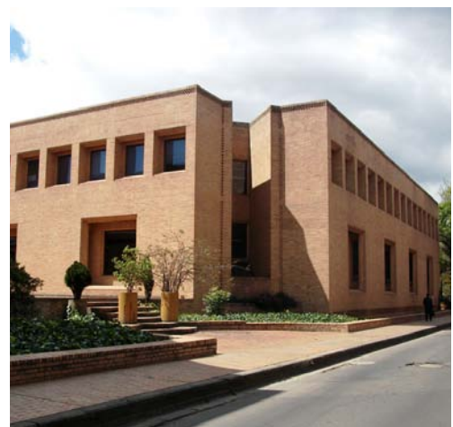
Deepness of the windows openings
