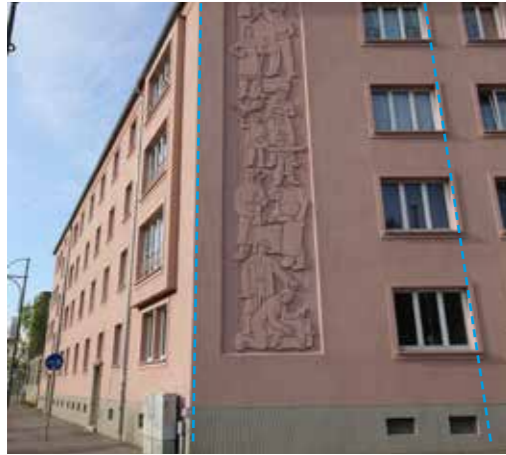
Picture before correction
