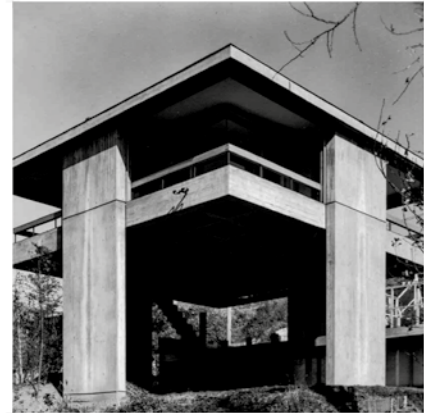
SKY HOUSE Kiyomori Kikutake's Sky House, 1958. "The house consists of a single 10x10m concrete slab raised up on 4.5 m high piers located on the central axis of each side, in order to free the corners."
