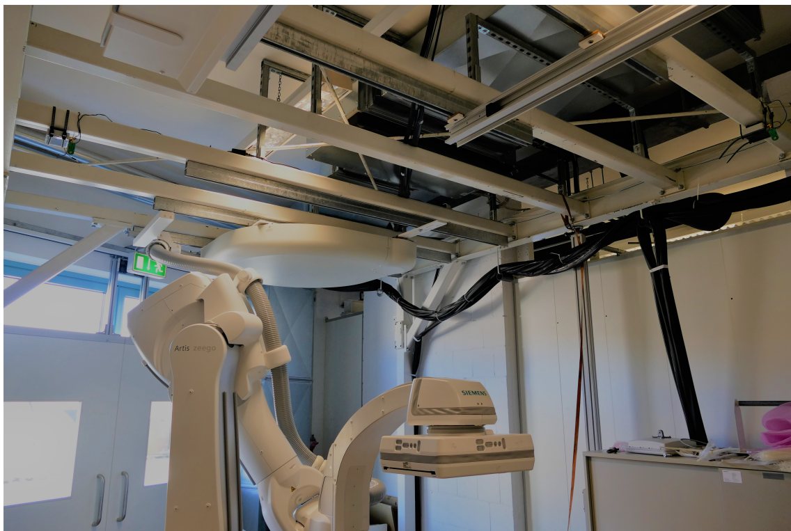
Figure 8.7: System setup for medical environment with two reference UWB anchors mounted at the ceiling.
