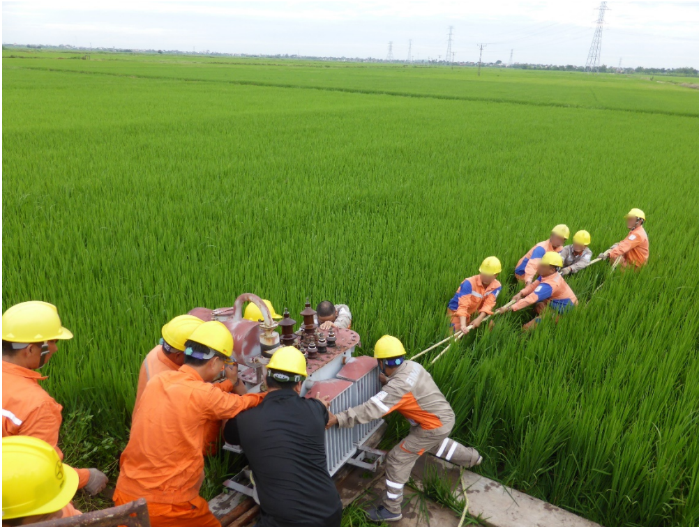
Figure 7. General Team Number Two relocates a transformer, summer 2019
