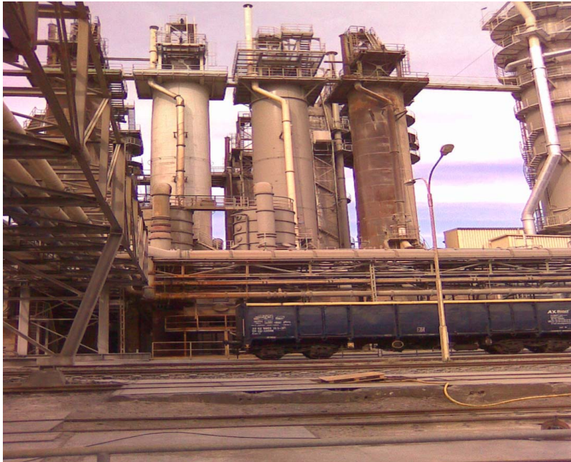
Figure 3.1: Mixed feed lime kilns.
