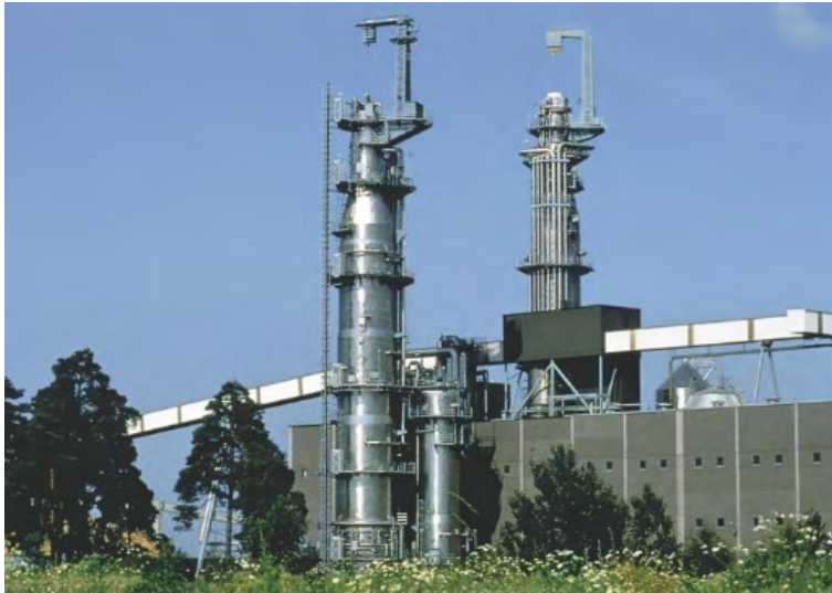
Figure 2-1: Standard 2205 duplex stainless steel continuous sulphate pulp digester and impregnation tower in Sodra Cell Mönsteras, Sweden.
