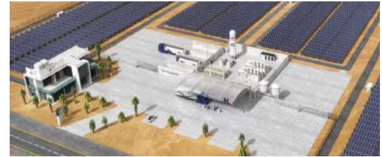
Cleanergy: H 2 Production & Refueling Plant
