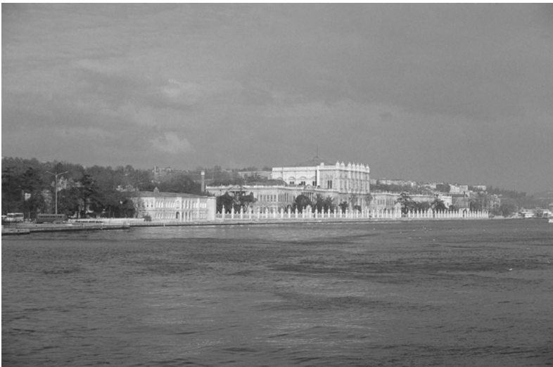
Fig. 5b: 1856: Dolmabahçe Palace. It is an example of an architectural style that the Ottomans were trying to adopt until the mid-19 th century.
