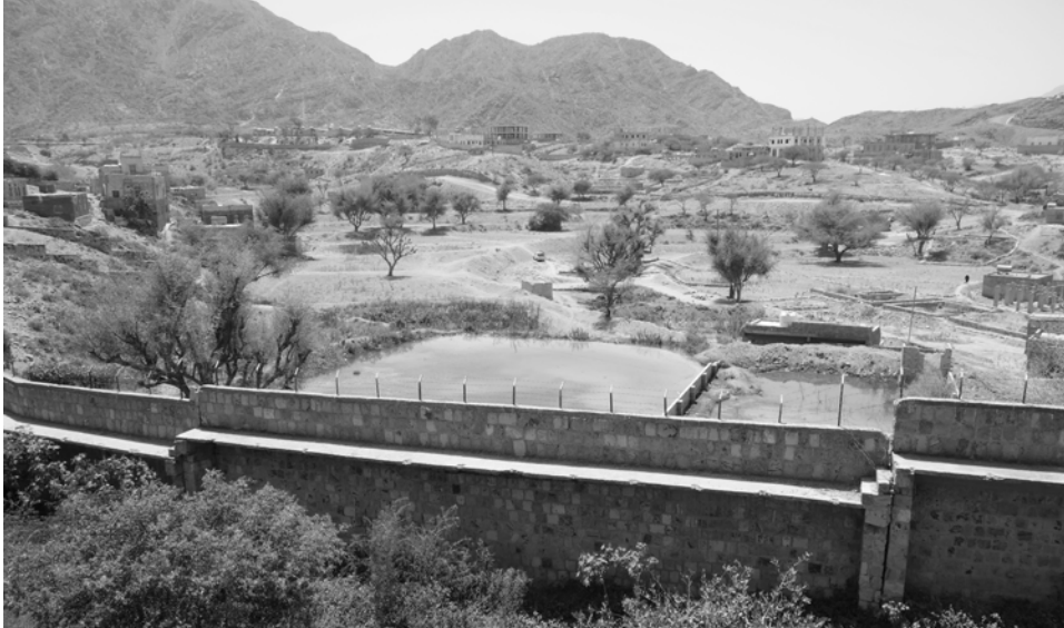
Photo 6. Sewage Leak Along Perimeter Wall, Taiz Central
