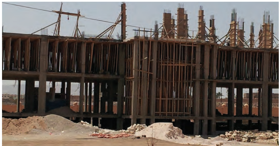
Photo 4. New judicial complex under construction in Taiz.
