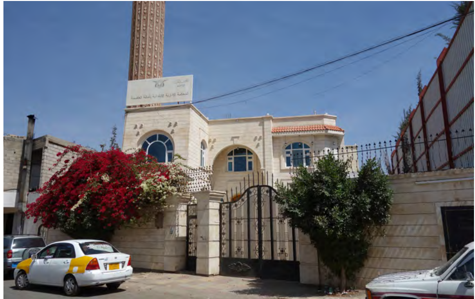
Photo A6.3 Special administrative court, Sanaa.
