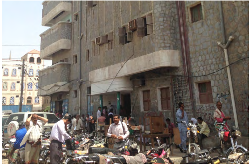
Photo A6.4 Hodeida North and circuit courts.
