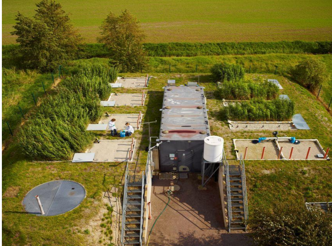
Figure 3.1-1 The pilot scale CW systems in Langenreichenbach: pairs of unplanted and planted with Phragmites australis subsurface flow CWs. Photo: André Künzelmann (UFZ); courtesy Dr. Jaime Nivala.
