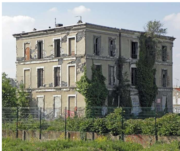
The first house built of reinforced concrete. By François Coignet, Saint-Denis near Paris, 1853
