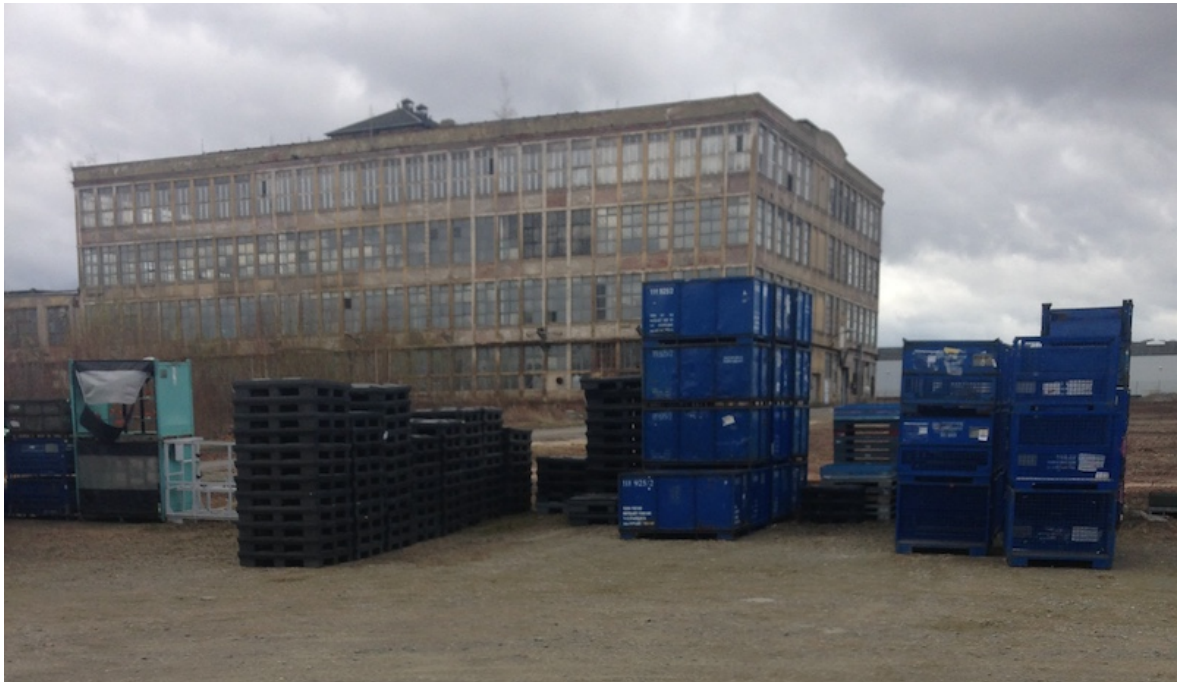
Figure 5. The preserved Sachsenring Werk I (former Horch) building.
