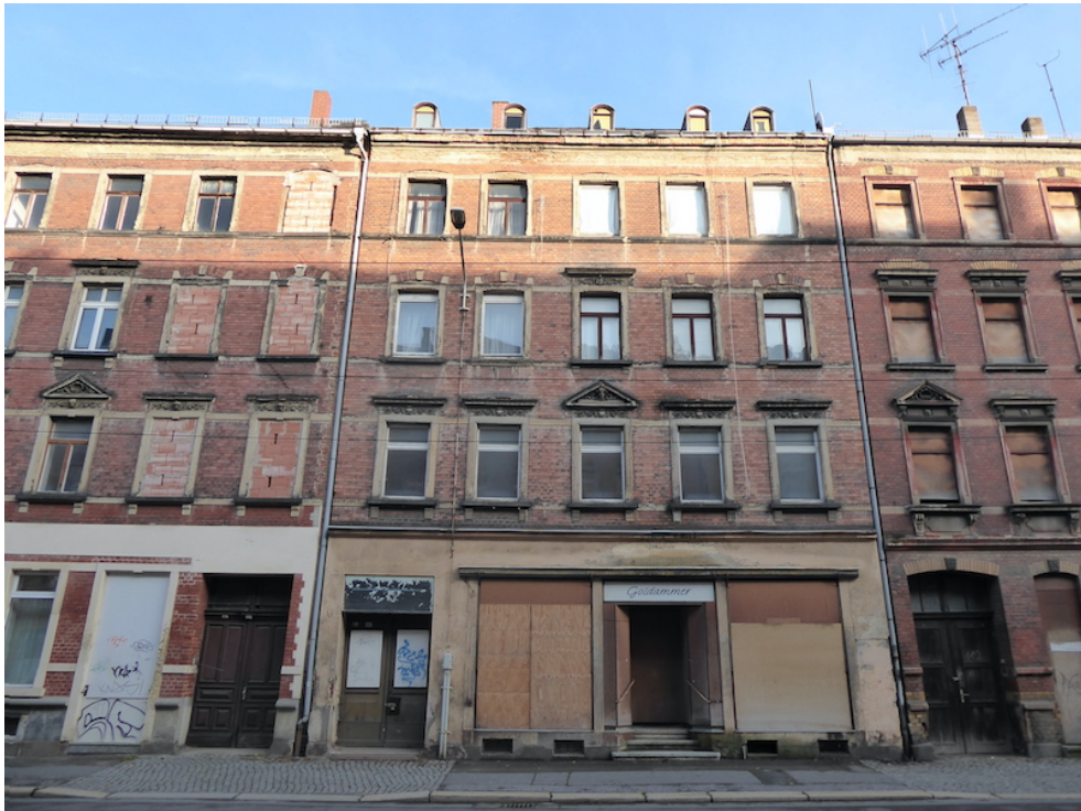
Figure 3. Empty houses on Zwickau's Leipziger Straße.
